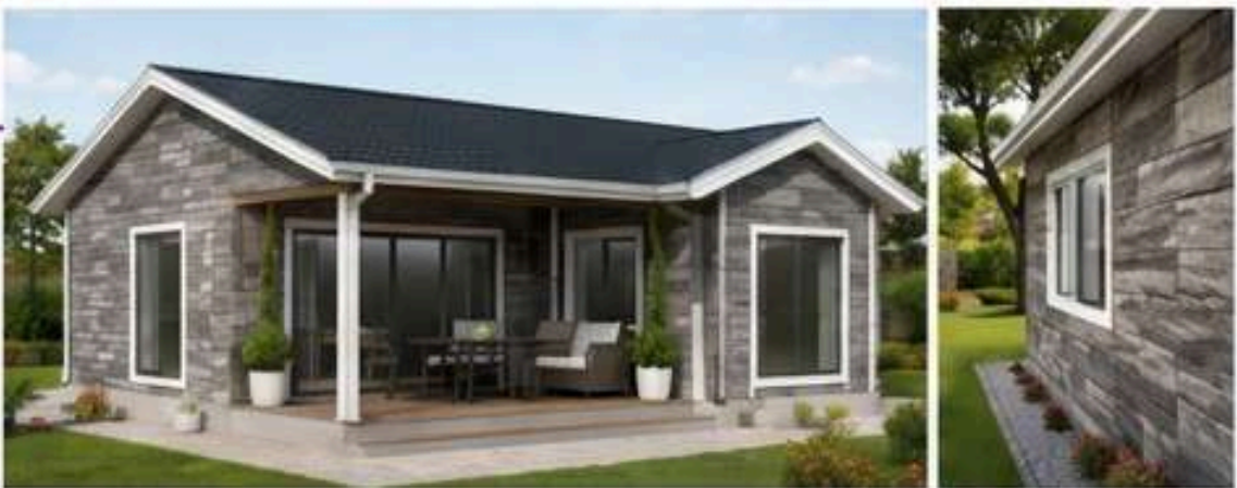
FINAL APPEARANCE STONE PATTERN CLADDING + PAINT Stone Pattern Clad Prefab House
